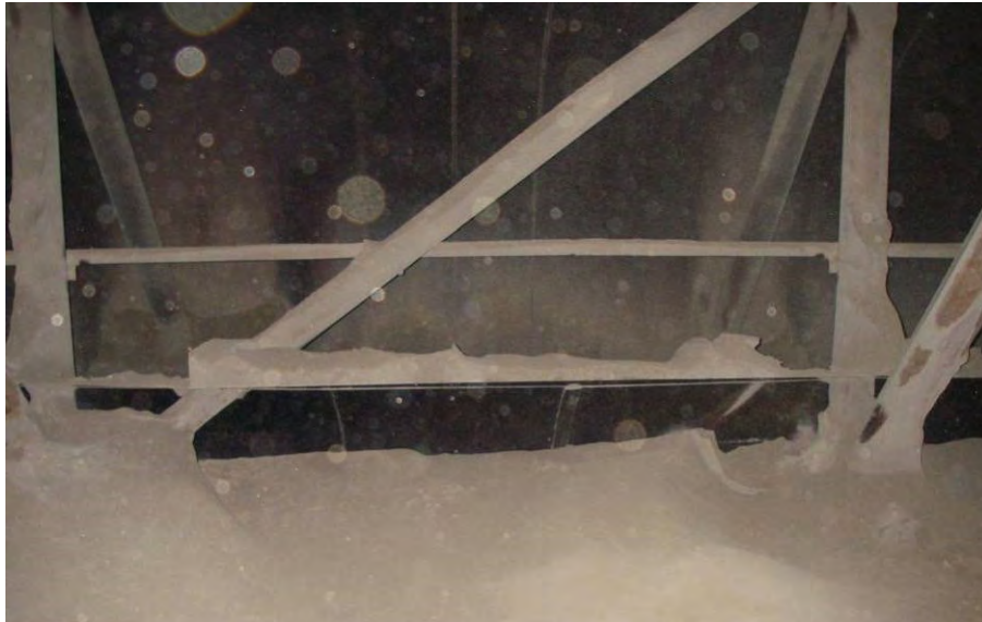
Still Have Ash Dropout in Crossover Duct
