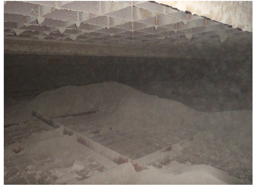
Smaller Ash Piles in L1-L3
