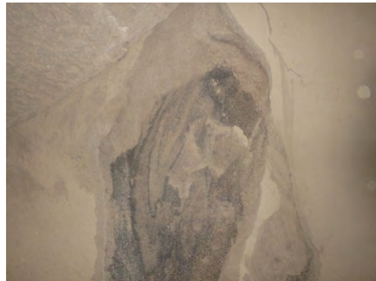
Unburned Carbon in Ash Piles
