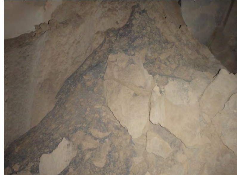
Unburned Carbon in Ash Piles
