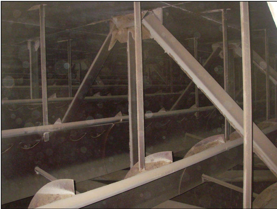
7 Reactor Hood Vanes “Clean” Condition
