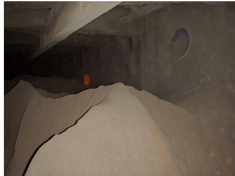
Ash Piles in L2
