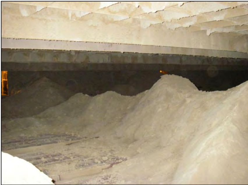
Larger Piles in L1-L3
