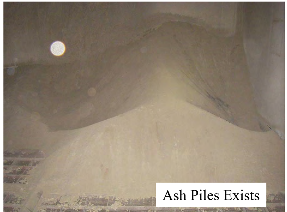
Still Have Ash Dropout in Crossover Duct
