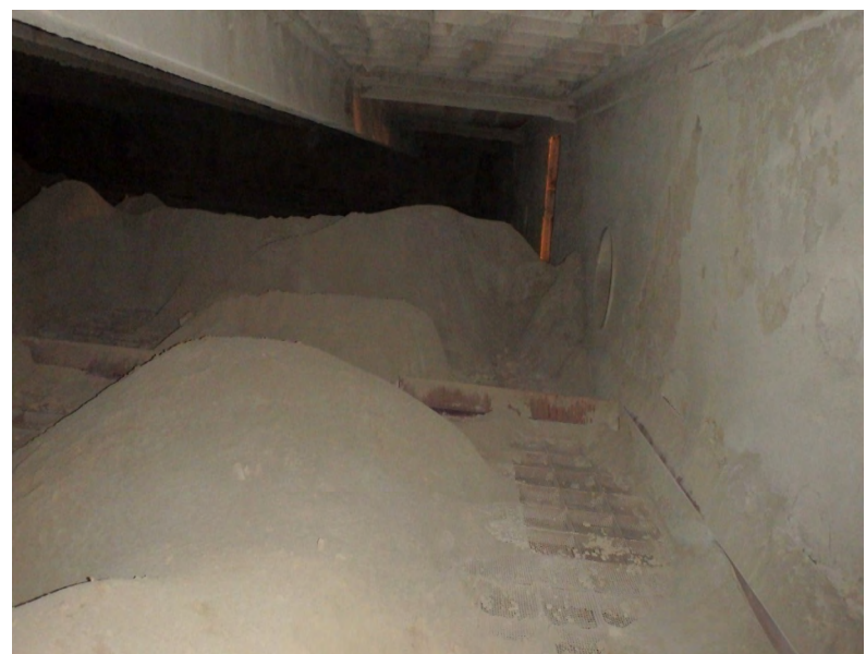
Larger Ash Piles From AIG to Far Side Through Center of Reactor
