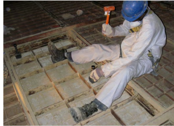
Mechanical Cleaning (Not Recommended)
