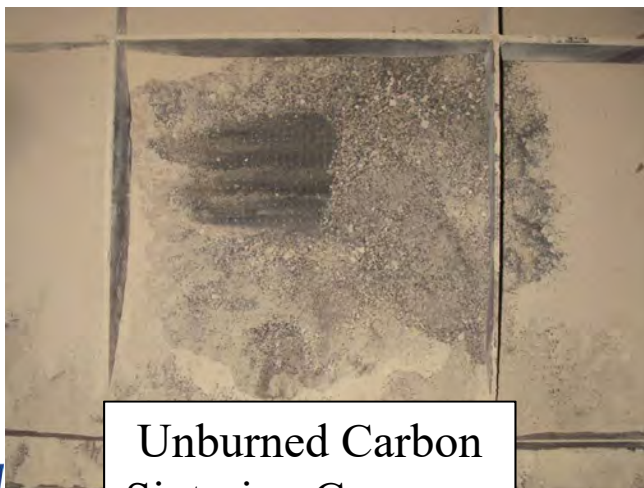
Still Have Ash Dropout in Crossover Duct
