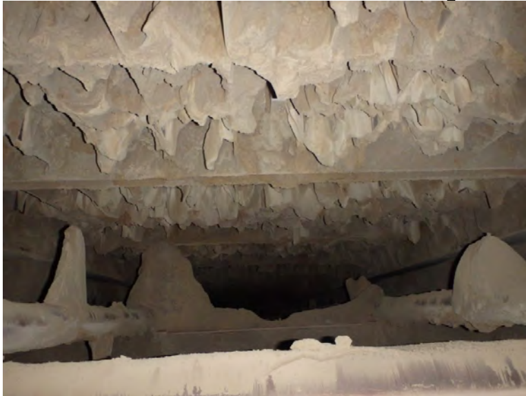
“Mud Daubers” on Outlet in L1
